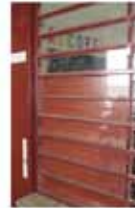
Picture 5: Adaptation not pursuant to the design: installation of plate on the frame so as to prevent break-ins (School "A") (Photo credit: A. J. G. Limongi França).
