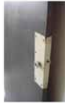
Picture 4: Adaptation in disagreement with the design: door made of iron sheet and heavy-duty lock (School "A") (Photo credit: A. J. G. Limongi França).
