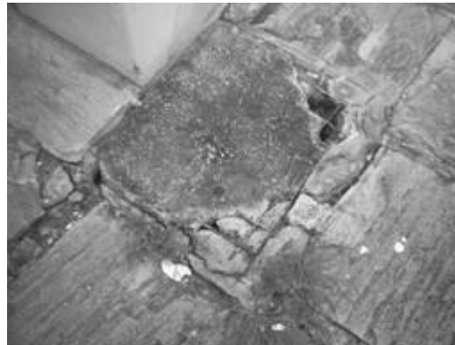
Figure 6. Septic tank with breaks and collapse in Building 05.
